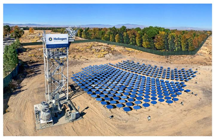
Heliogen says the intense heat from its solar operations can be collected and processed to generate electricity, power industrial processes or produce hydrogen fuel—even when the sun goes down.
